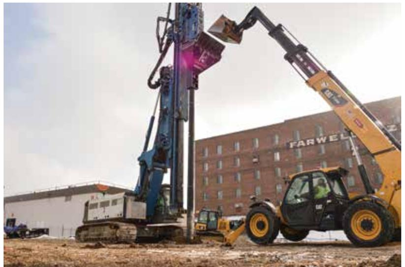
Above: Our DeepFeed VSC system is a direct-push, bottom feed installation method and allows the vibratory stone columns to be pushed to depths of more than 40 feet. Shown at a multi-family Apartment Building site in St. Paul, MN.
