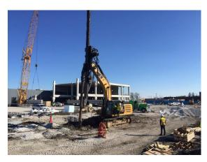
showing topsoil, Vibratory Stone Columns (VSCs) were an acceptable method. There were about 350 linear feet of strip footings and several column pads, so VSCs were recommended as an economical alternative to undercutting the soils under the footings.
